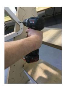
**1.1** Place the handrail modules on the outer stair stringer of the folding staircase so that they are each in the middle of a stair stringer element. It is recommended to start at the staircase exit to create an even distance between the handrail modules.
