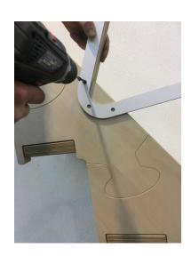
**1.1** Use the pre-drilled holes in the handrail module to transfer the holes to the outer stringers of the staircase. A screw clamp can be used to prevent the modules from slipping during drilling. Use a 9mm wood drill bit to drill as straight as possible from both sides halfway through the stringboard to ensure a perfect fit.
